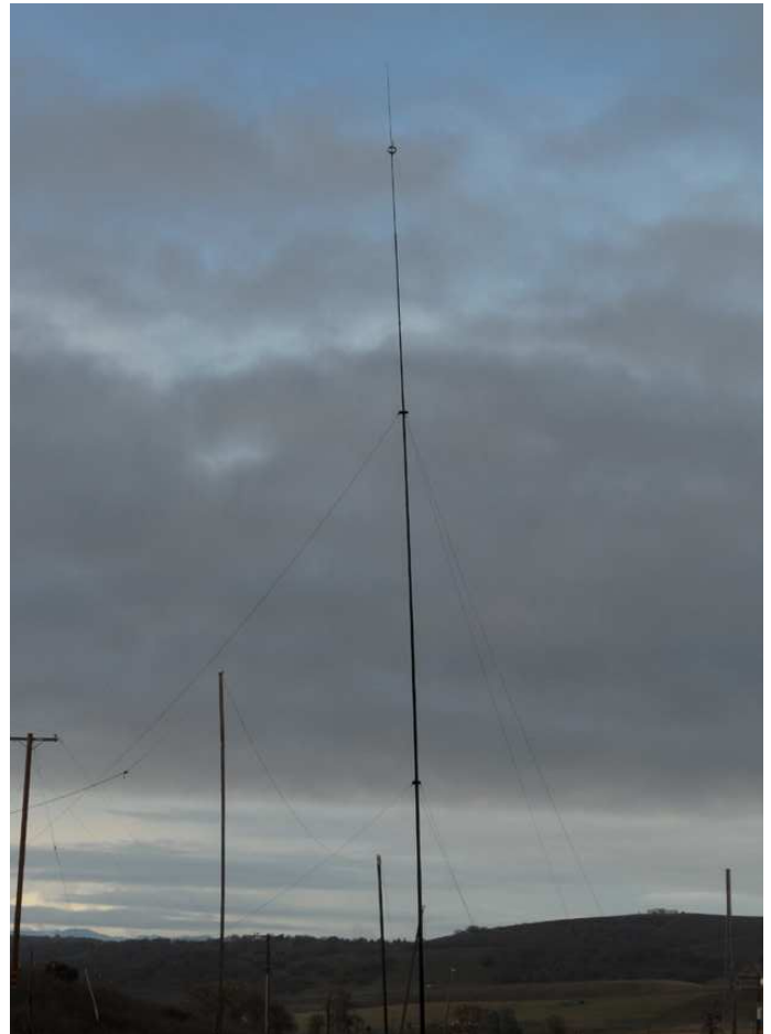
The antenna and support poles for the elevated radials.
