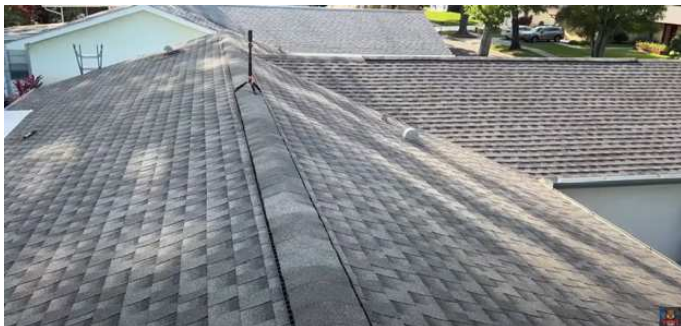
Bob, KD4BMG, tucks the elements of an off-center-fed dipole antenna into the roof vents of his home.
