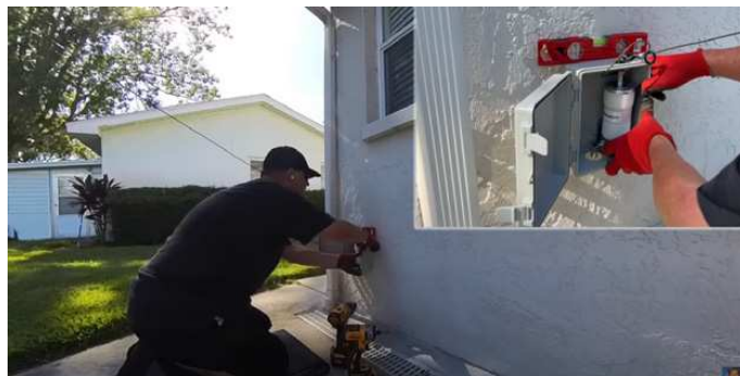
Bob, KD4BMG, installs Chameleon Antenna hardware on the wall of his home in a stealth antenna setup.
