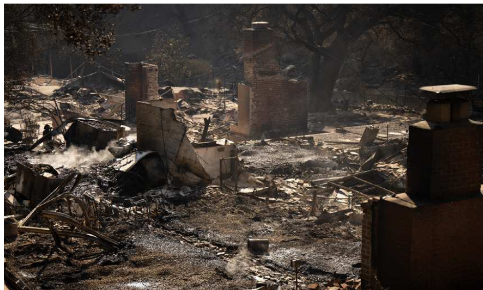
Damage from the Eaton fire in California. [US Air National Guard photo]
