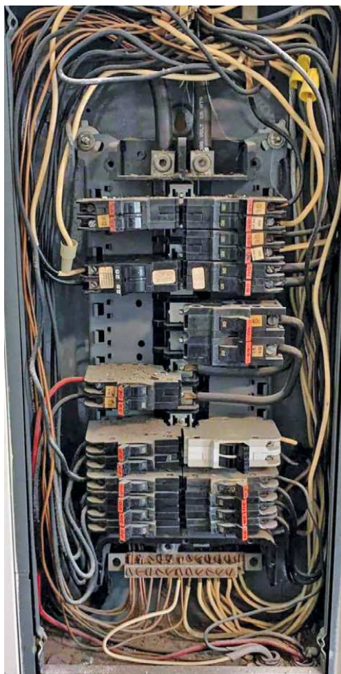
Figure 1 — An example of a split bus panel. These panels contain two separate sets of bus bars. [www.waypointinspection.com]
