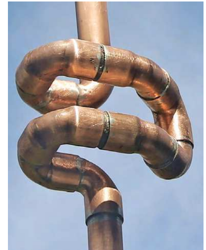
Figure 3 — The assembled phasing stub.
