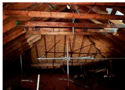
The author's attic antennas. His three-element, 6-meter beam is in the middle. If you look closely, you can see his two 20-meter dipoles and 6-meter loop.
