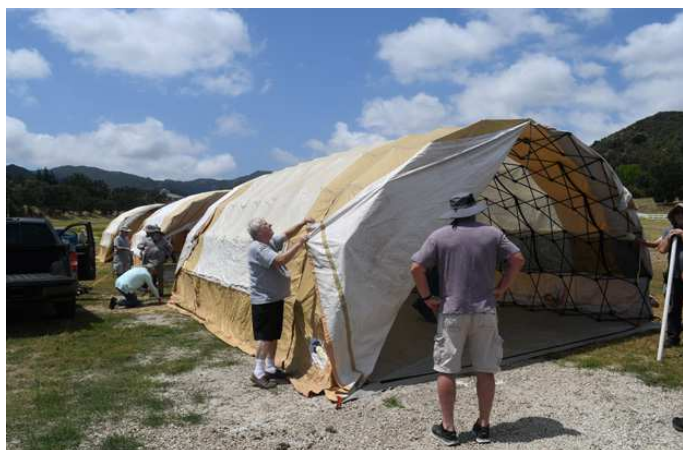
CVARC members erecting emergency operations tents on the eve of ARRL Field Day.
