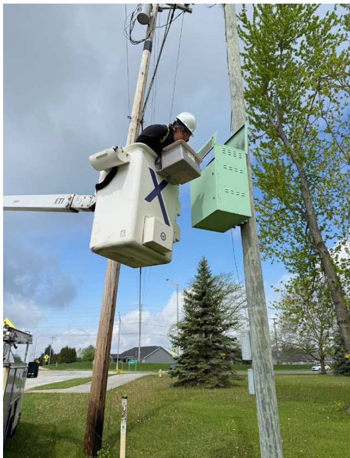
Cable company technician analyzing the suspected source of the RFI. [Carl Luetzelschwab, K9LA, photo]
