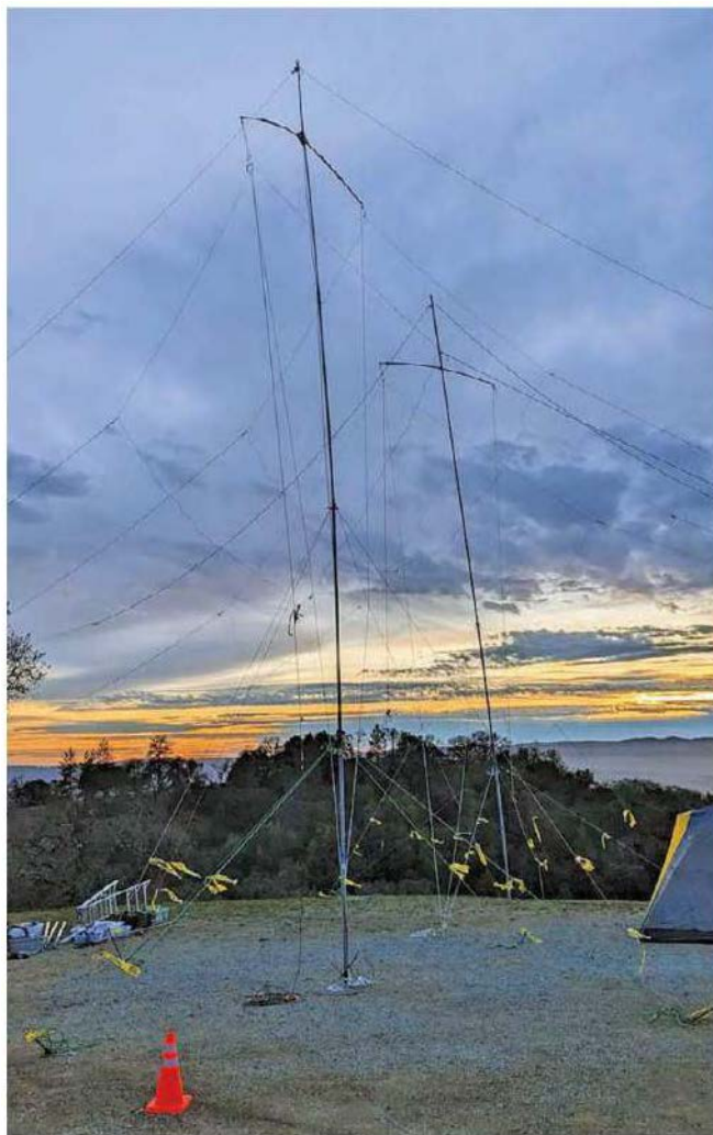
Figure 1 — Use yellow or orange safety tape to flag all of the guy lines, and place traffic cones to keep vehicles in a safe place. [Steve Sergeant, KC6ZKT, photo]
