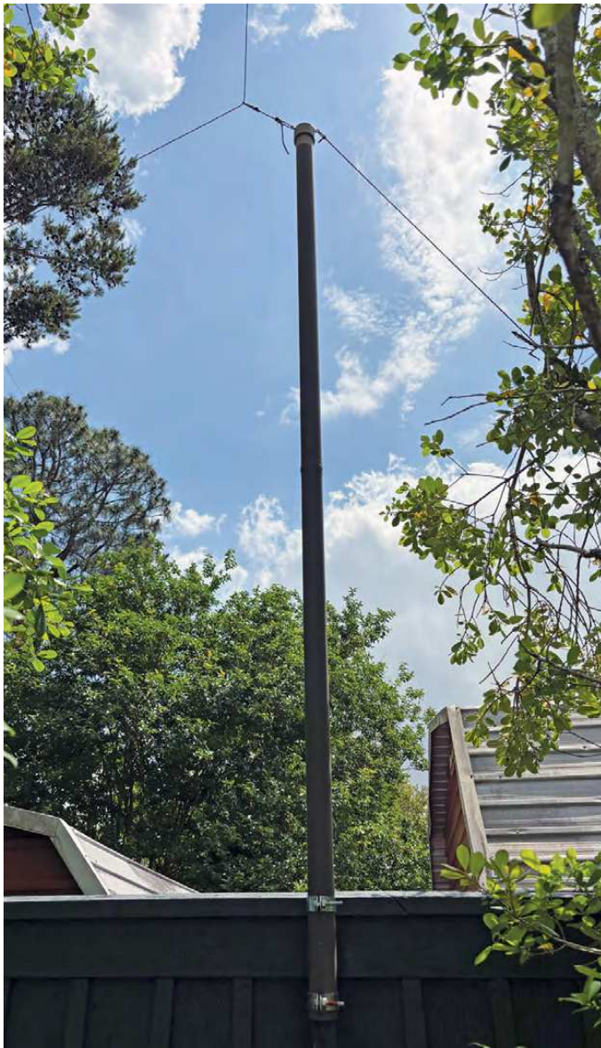
Hurricane Ida damaged the wooden post holding Brian Karcher's, KG5GJT, end-fed antenna, so he replaced it with a fiberglass military tent pole. [Brian Karcher, KG5GJT, photo]
