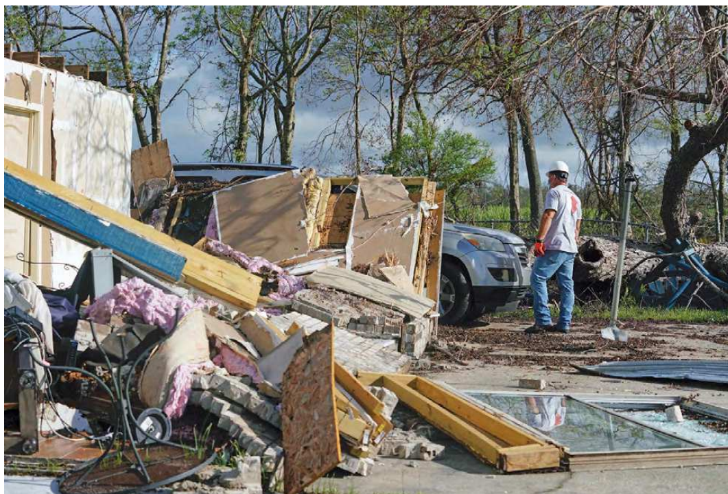
Damage is assessed in Hahnville, Louisiana, during the aftermath of Hurricane Ida. This was about 25 minutes away from Brian Karcher's, KG5GJT, home. [Photo courtesy of FEMA]
