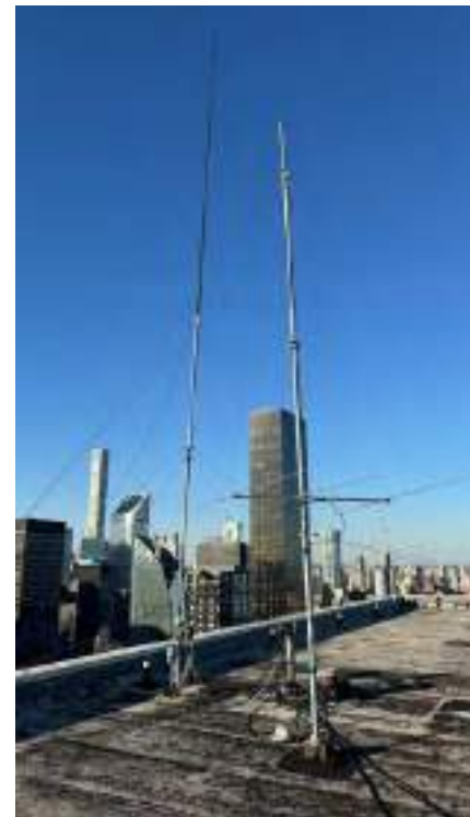
Antennas for 4U1UN on the roof of the UN Headquarters. The main antennas are a SteppIR BigIR vertical and an inverted-V dipole. [Adrian Ciuperca, KO8SCA, photo]
