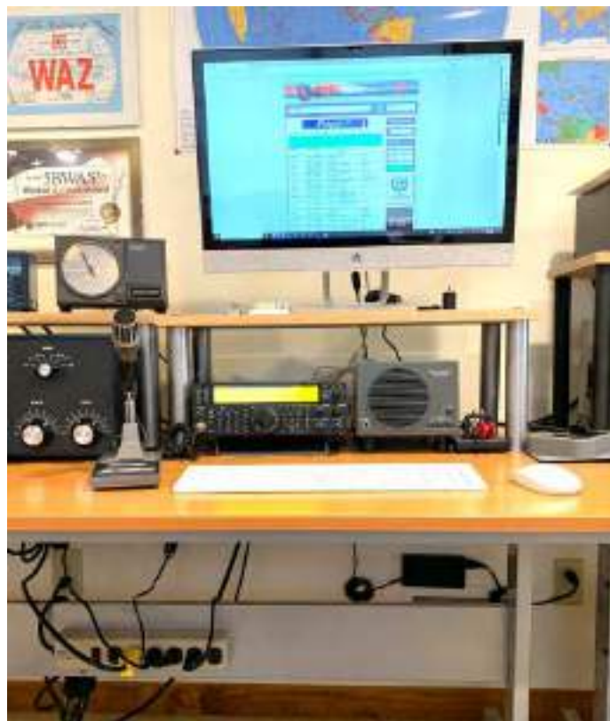
Figure 1 — The power supply brick mounted to the wall and away from any coaxial, audio, or control cables. [Scott Freeberg, WA9WFA, photo]
