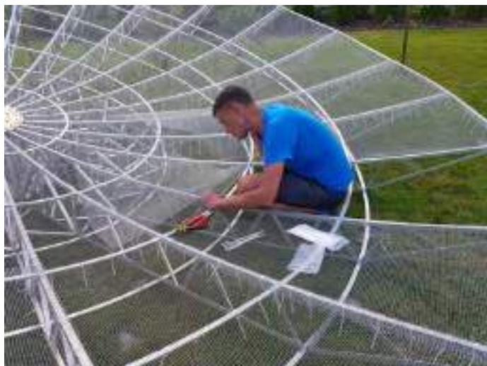
Figure 2 — Rafael fixes the last pieces of reflective metal mesh to the dish's aluminum frame.
