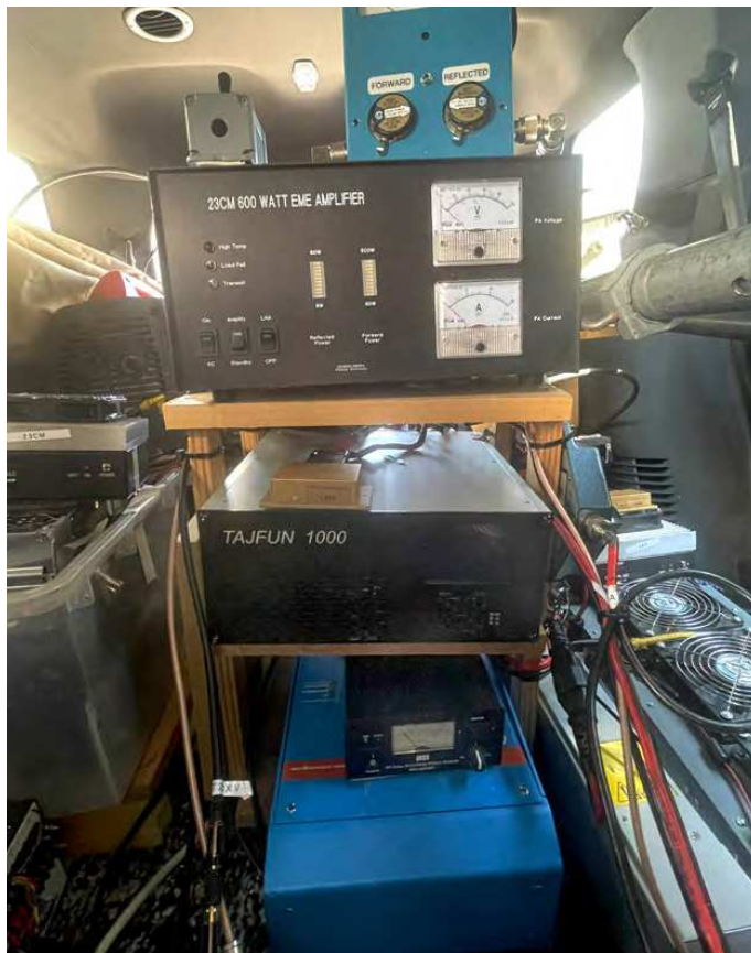
Figure 3 — The station's power amplifiers, which replace the back seat of the vehicle.
