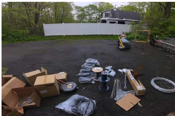
Ray, W2RE, shows some of the additional equipment needed for a successful installation of a tower and antennas.
