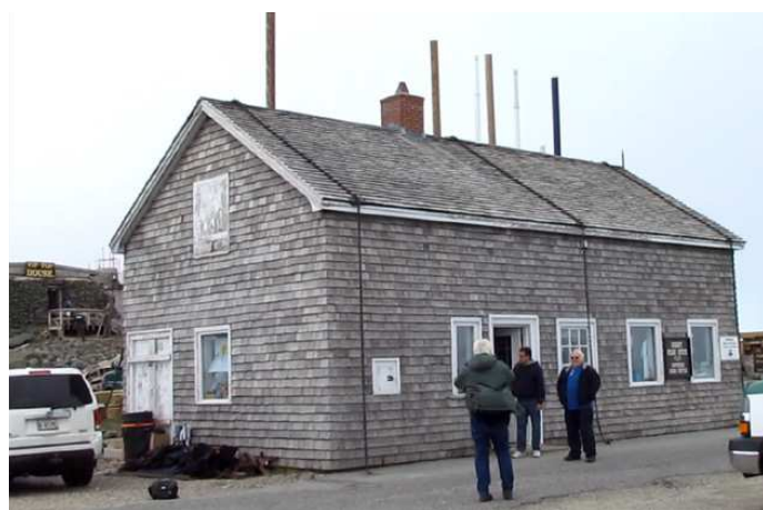
Figure 1 — Dave Olean, K1WHS; Tom Cefalo, W1EX, and Don Twombly, W1FKF, after installing the 10 GHz beacon inside the building on Mount Washington in New Hampshire. The cylinders on top of the building are radomes with antennas inside. [Paul Wade, W1GHZ, photo]
