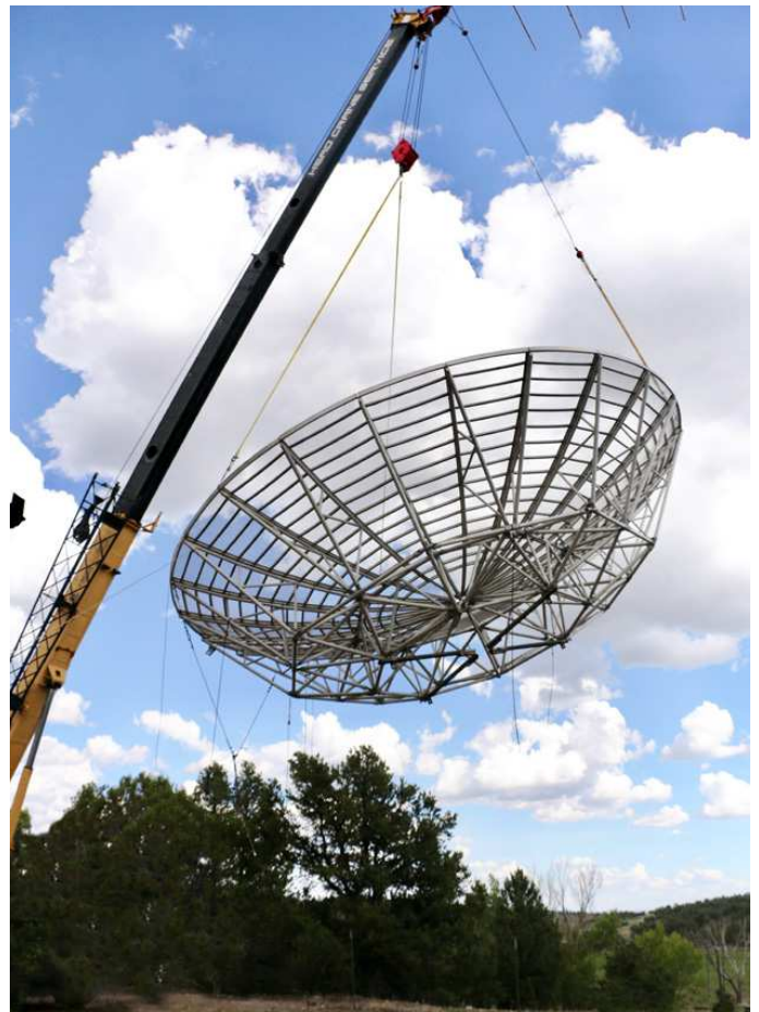
The dish lifted in the air by a crane and rotated to the birdbath position while being lowered to the ground.
