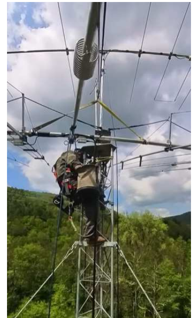
Ray, W2RE, working on an antenna installation at a height of 75 feet.
