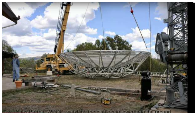
Chas Barrett, WDOC, watching the dish being lowered to the ground.
