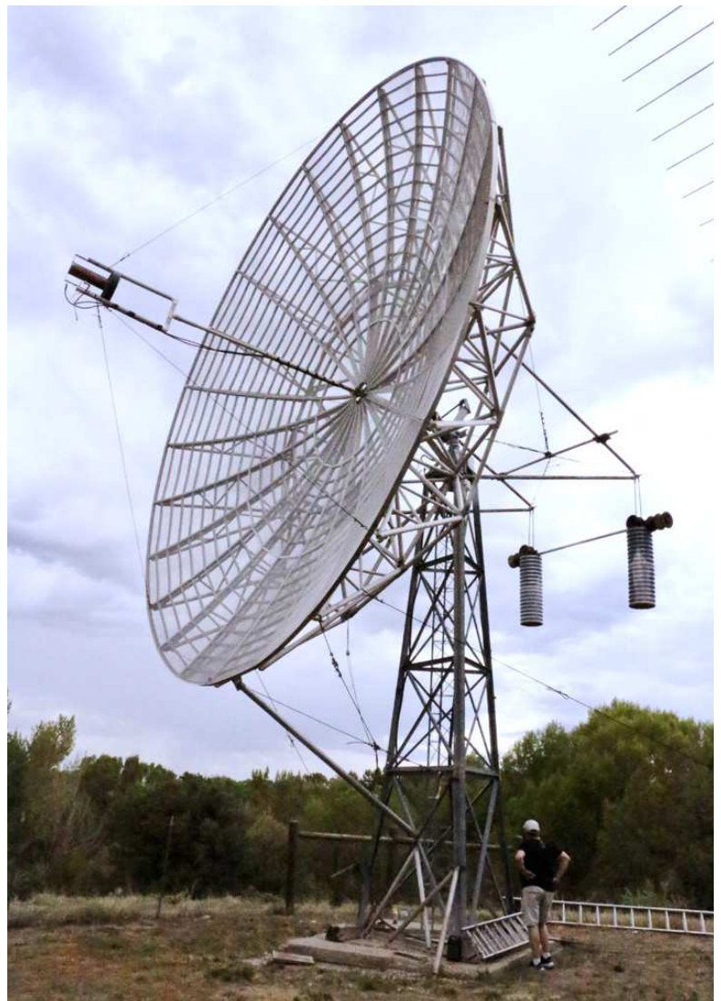
The 30-foot dish in the sideways position. This position presented the first challenge to the crew and the crane operator.
