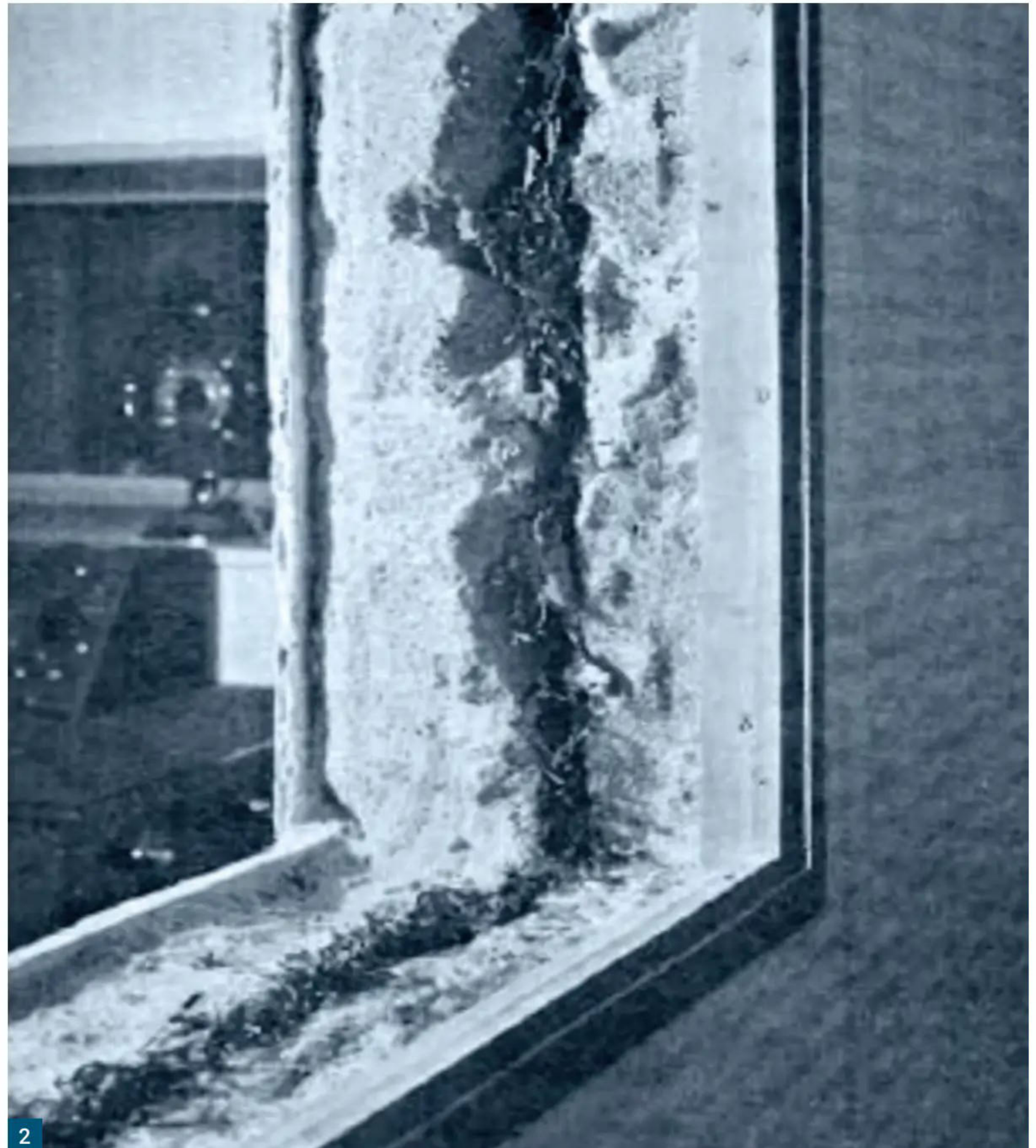
Fig. 2: An example of a specially constructed sound-proof window featuring eel grass sandwiched between walls of pumice concrete.
